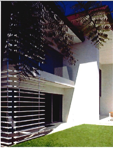
1 BAGGED & PAINTED MASONRY
